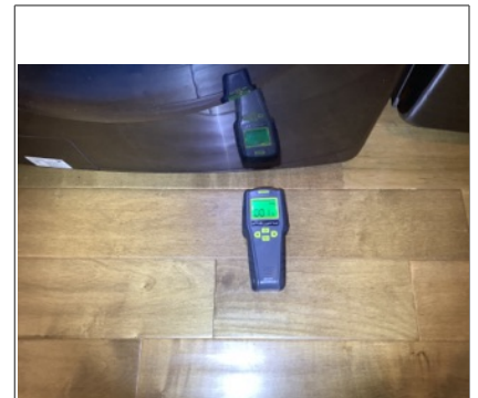
Moisture levels at the subfloor in the laundry room appeared to be within a normal range at time of inspection unless noted. Moisture levels were observed utilizing a pinless moisture meter.
