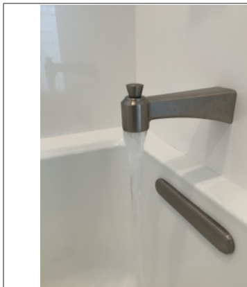
No active water leakage was apparent at time of inspection unless noted.
